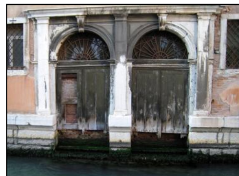
Crumbling Venetian building. Porous stucco must be used for renovation. In Venice's damp conditions everything else tends to fall off in sheets causing a hazard to passers-by.
